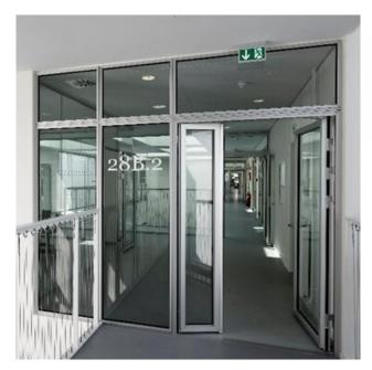
The photo shows an example of the glass wall system ID85, with or without fire rating, there is no visual difference.
