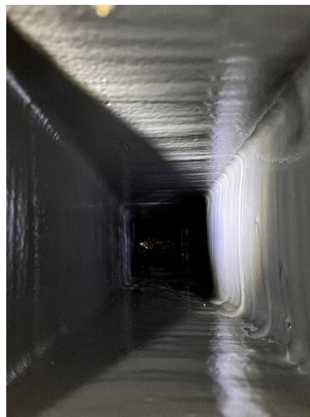
Figure 4 - Declared product, VC50, applied on ventilation duct of fiber cement.
